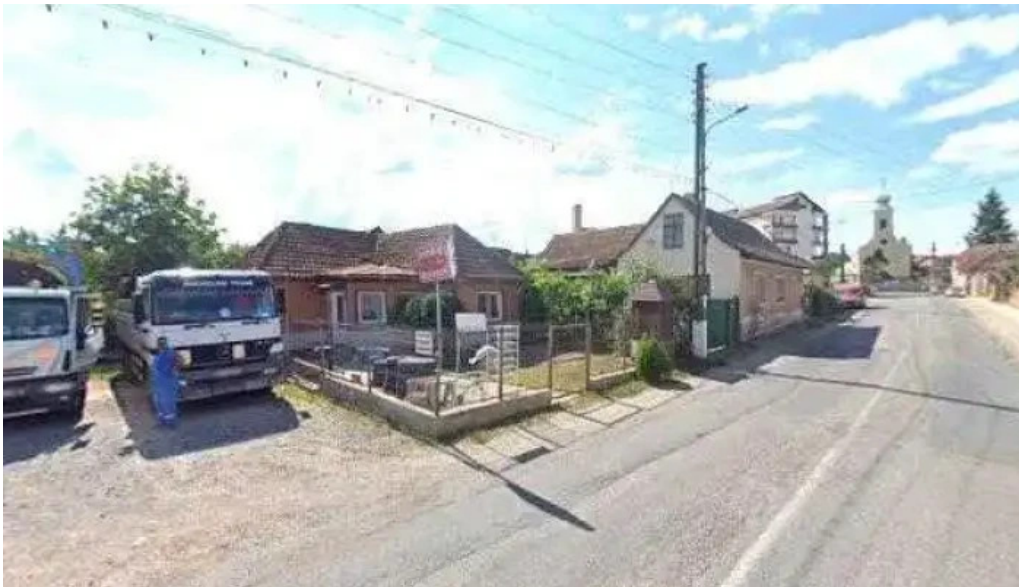
Restaurant pensiune barcaul street view si 360deg
