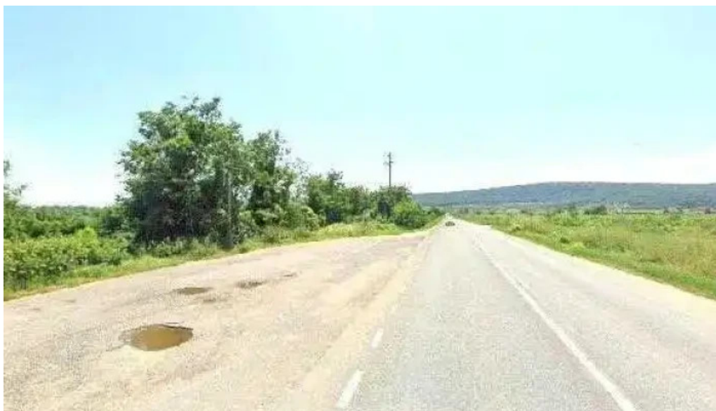
Restaurant ioba camping miraslau street view si 360deg
