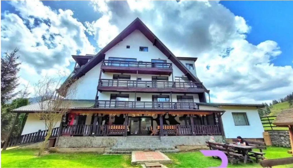
Green house podu dambovi?ei
