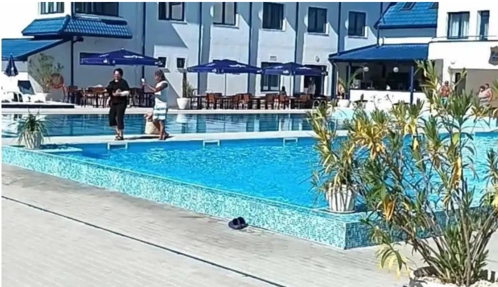
Complex balneo termal vata bai exterior
