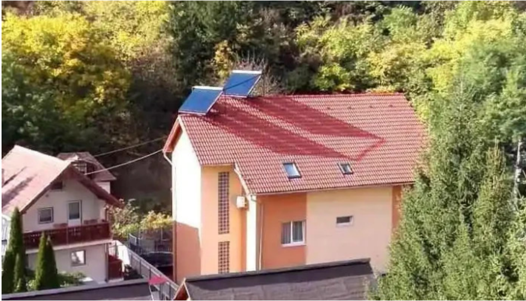
Hotel vacanta exterior
